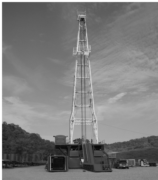
Figure 2-16. Typical Drill Rig with Derrick
