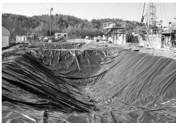
Figure 2-18. Lined Mud Pit
