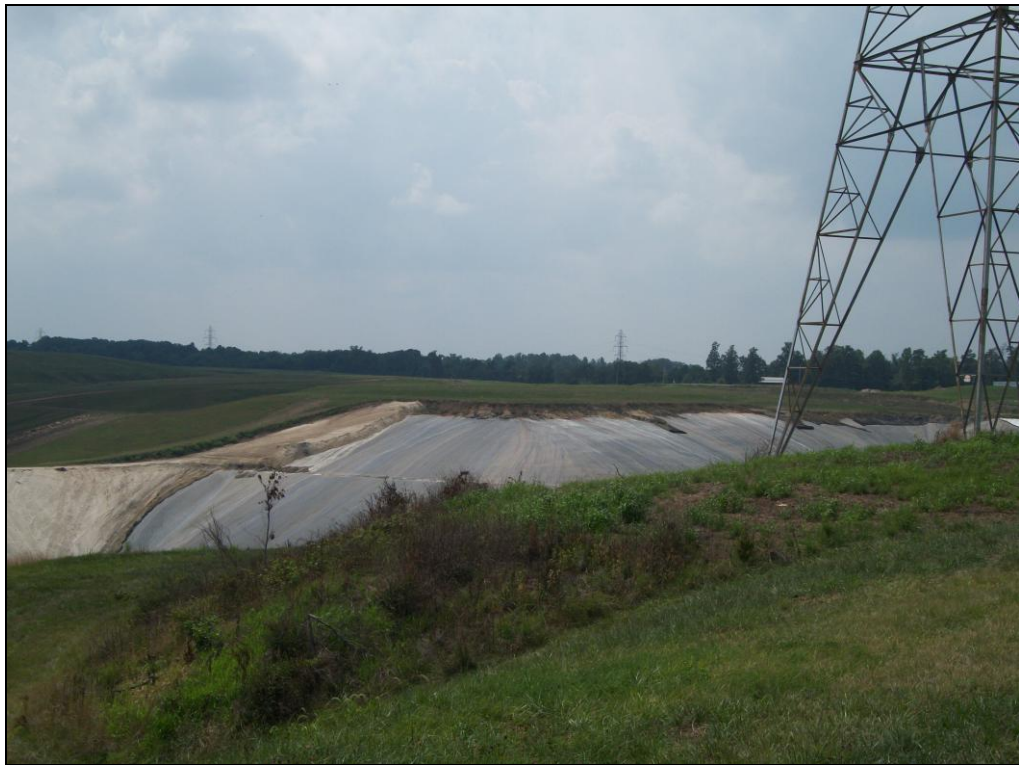
Photo 2. Ash and gypsum disposal cell within Little Broad Run landfill, showing general disturbance conditions; view to southwest.
