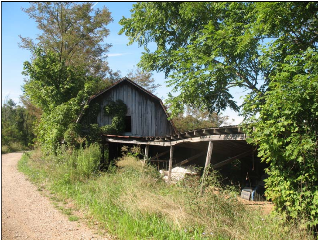
MS-0164: Barn and Tractor Shed, looking south
