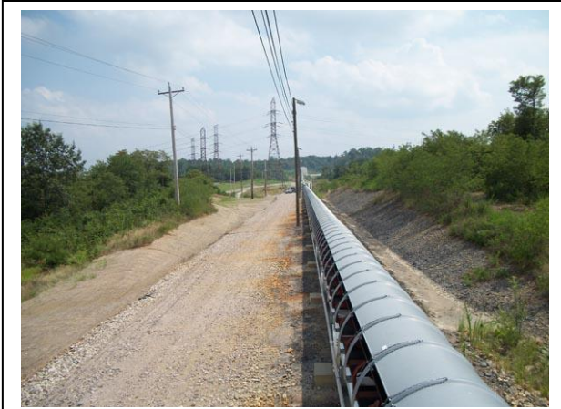
Figure 5-1. View to the south of the existing conveyor system running through the North Corridor project area, showing associated ground disturbance.
