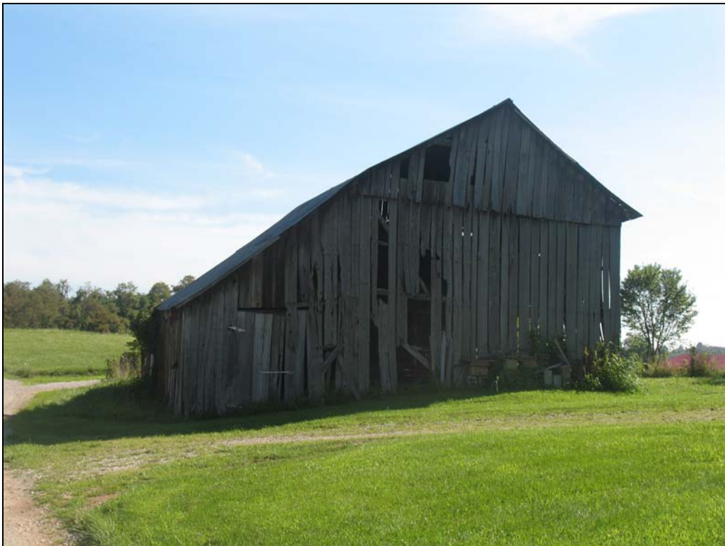
MS-0163: Durst House Barn, looking north
