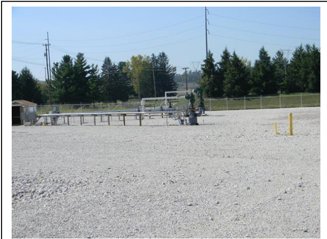
Figure 5-29. Existing conditions at the potential Mountaineer Plant well site, showing extensive ground disturbance; view to southwest.
