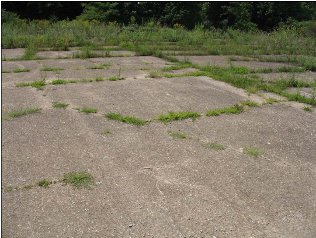
MS-0173: Slab Foundation, looking southwest
