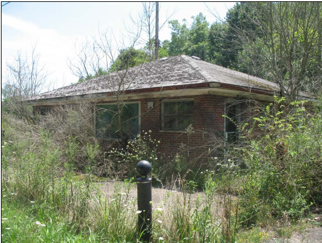
MS-0169: Brick Building, looking southeast
