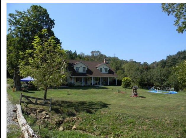
Figure 5-18. Small floodplain of West Run and adjacent domestic structure present in the southern portion of the East Corridor; view to the southeast.
