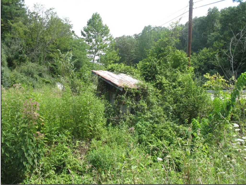
MS-0166: Outbuilding, looking northeast
