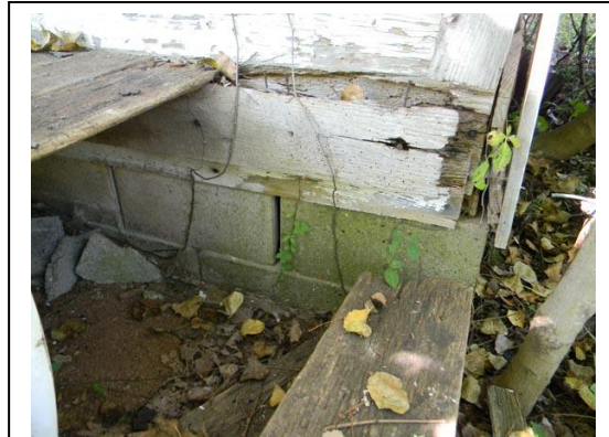
Figure 5-35. View to the northeast of abandoned modern house cinder block foundation (MS-0164).
