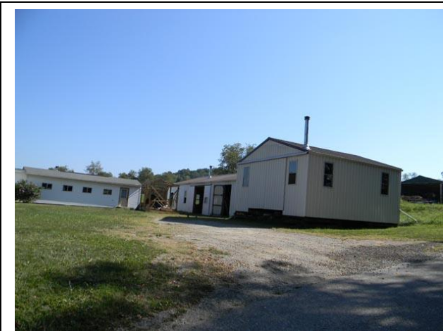
Figure 5-14. View of domestic structure and associated ground disturbance present within the western portion of the Foglesong Corridor.
