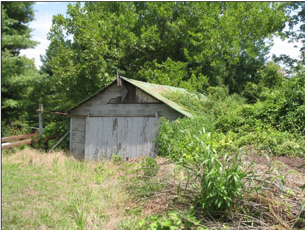
MS-0174: Garage, looking northeast
