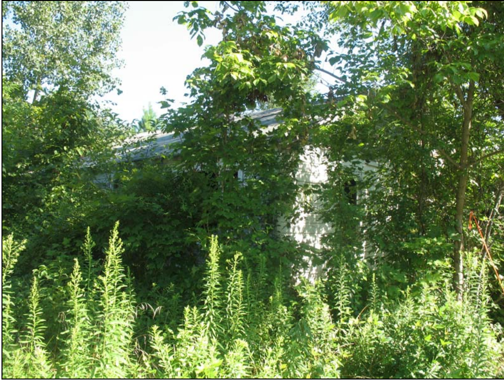
MS-0164: House, looking northwest
