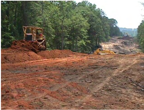
Clearing and Grading
