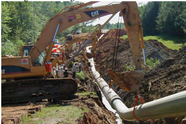
Laying Pipe and Backfilling
