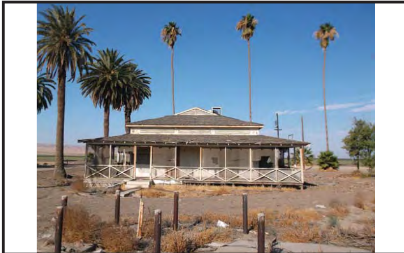
Adohr Farms/Palm Farms Foreman's Home and Office (Building B)
