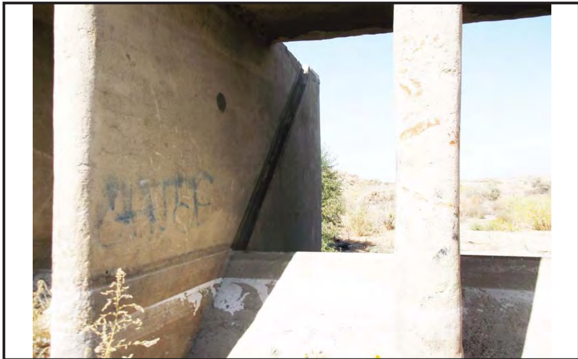
Old Headquarters Weir- View of Channel for Flashboards
