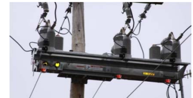
Smart switches help ensure grid reliability and power quality
