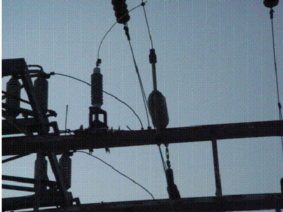
Figure 6: Granville Station, HV-BPL Coupler
