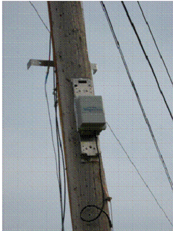
Figure 13: BBU Battery Backup System
