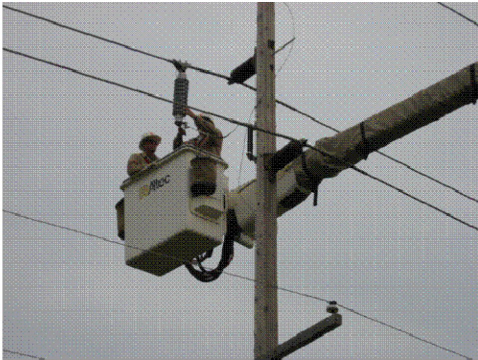
Figure 10: Installing T-Line RF Coupler at Pole 41
