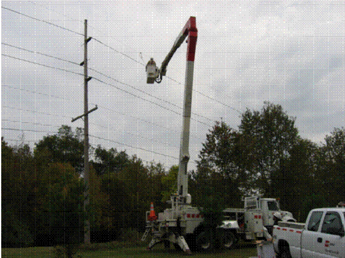
Figure 9: Start of installation at Pole 41.
