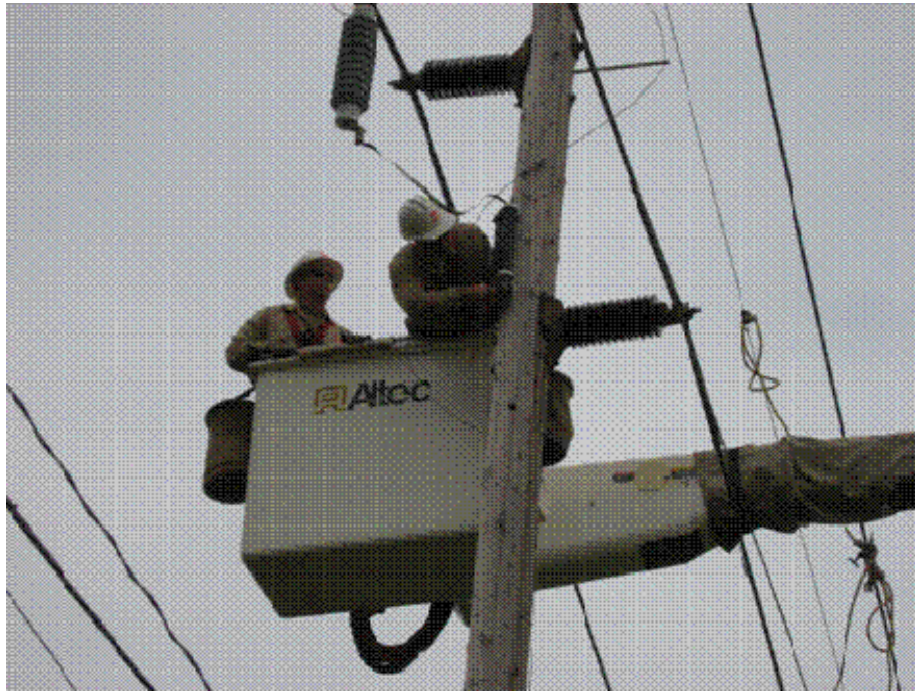
Figure 11: Installing T-Line RF Coupler at Pole 41
