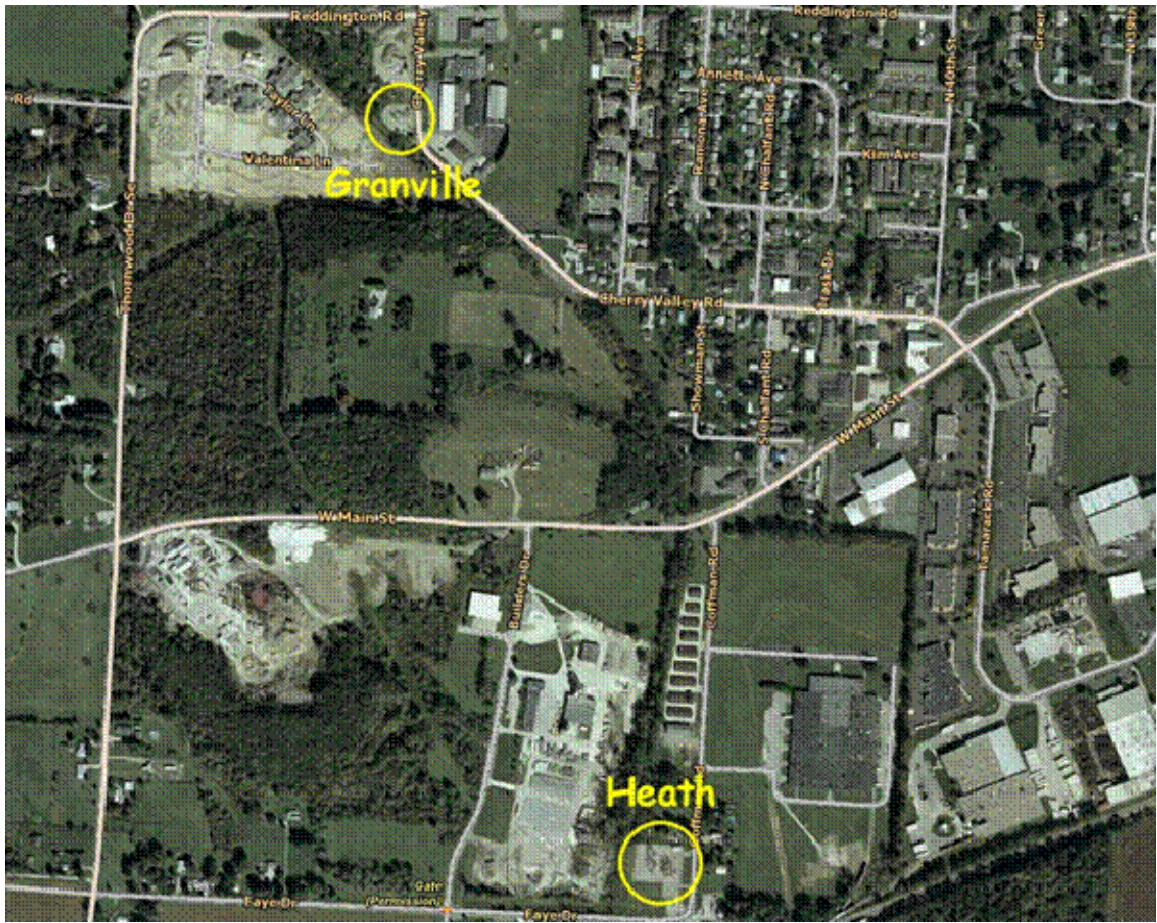
Figure 3: Heath and Granville substations in Newark Ohio
