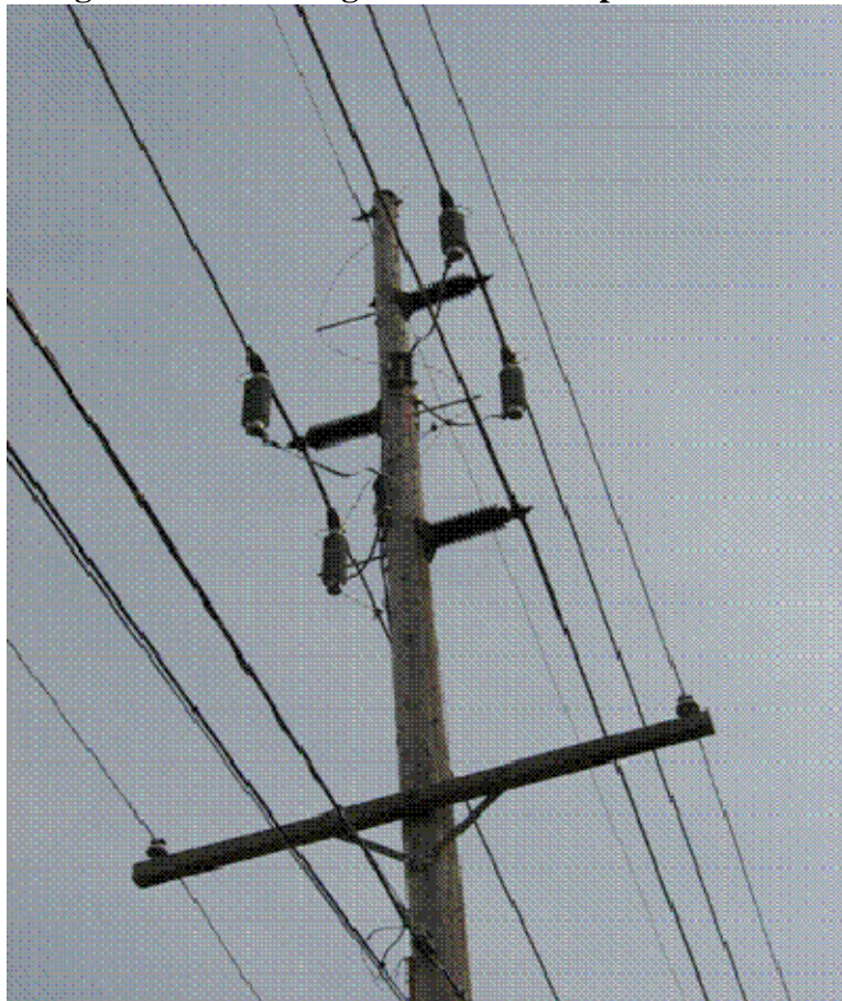
Figure 12: (4) T-Line Coupler Installed at Pole 41
