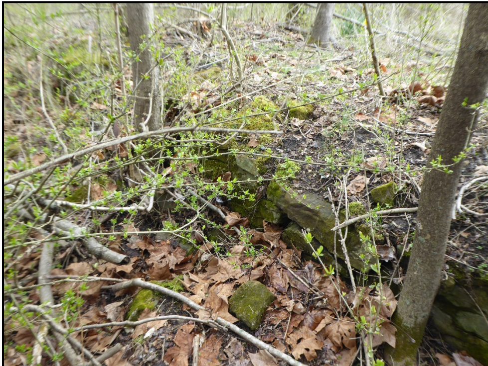
Figure 34: East foundation wall, facing north.
