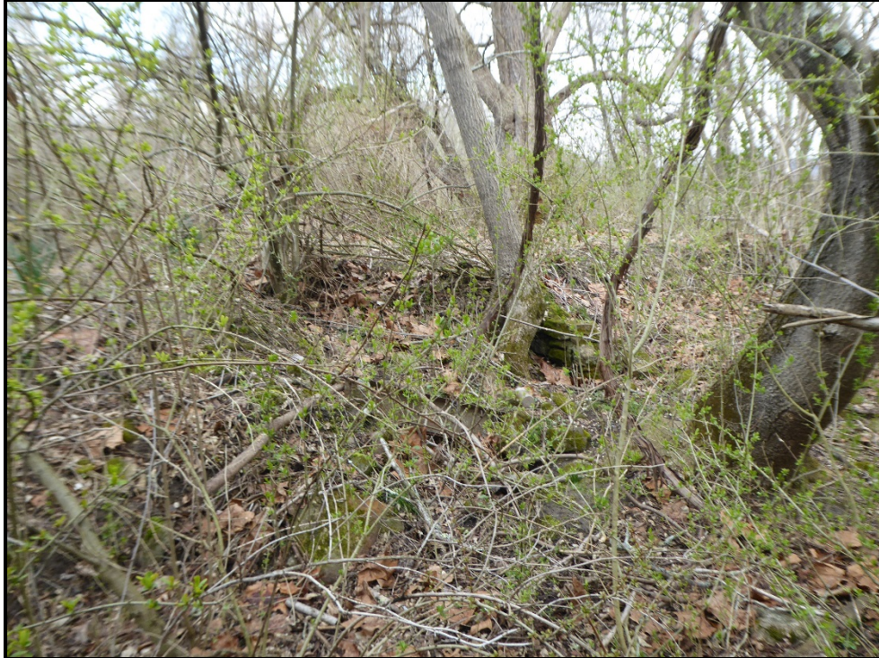
Figure 37: Foundation interior, facing west.
