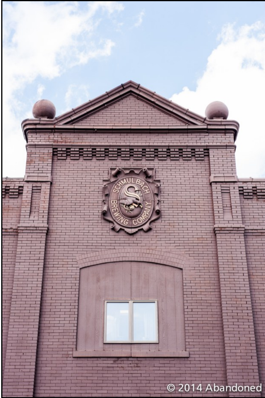
Figure 48: Portion of the abandoned Schmulbach Brewing Company building in Wheeling, West Virginia (courtesy abandonedonline.net).
