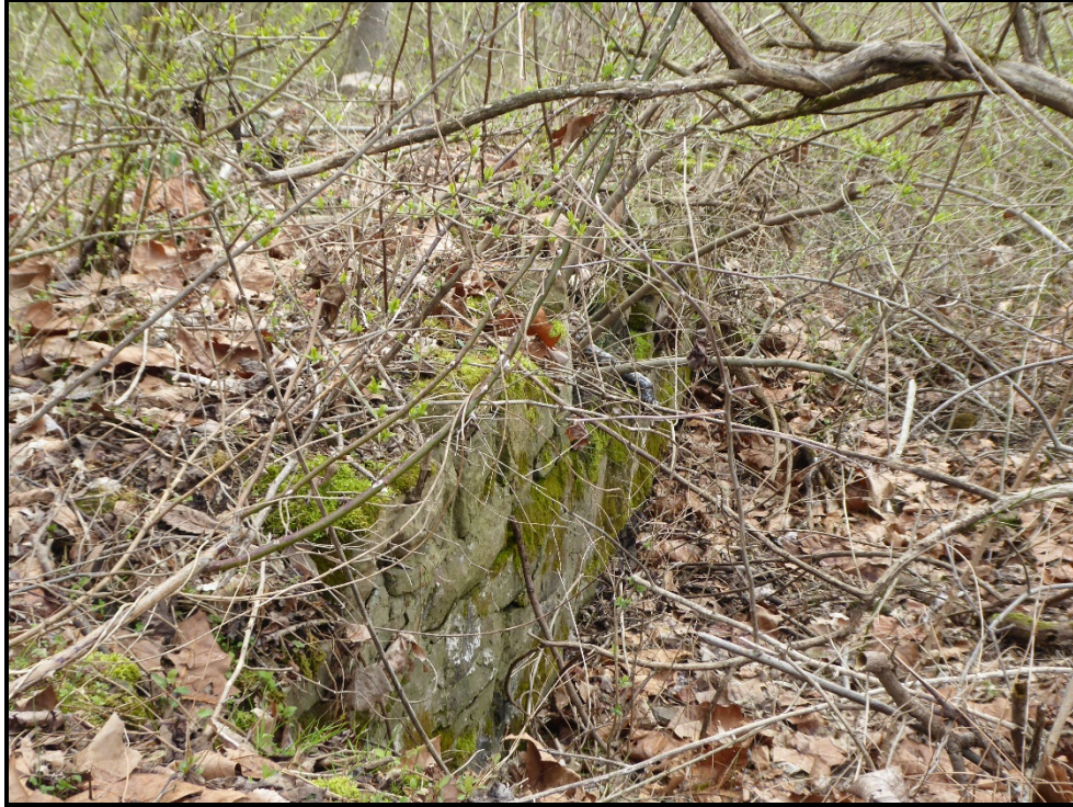
Figure 35: South foundation wall, facing southwest.
