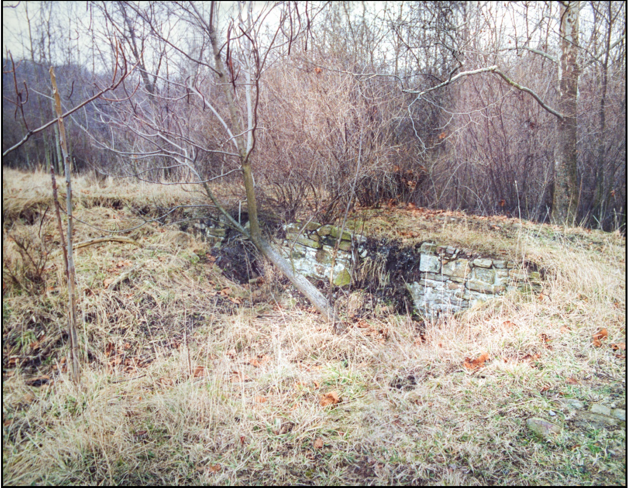
Figure 13: Stone foundation as it appeared ca. 1991, at the time of the Ecology and Environment, Inc. survey (courtesy NETL).
