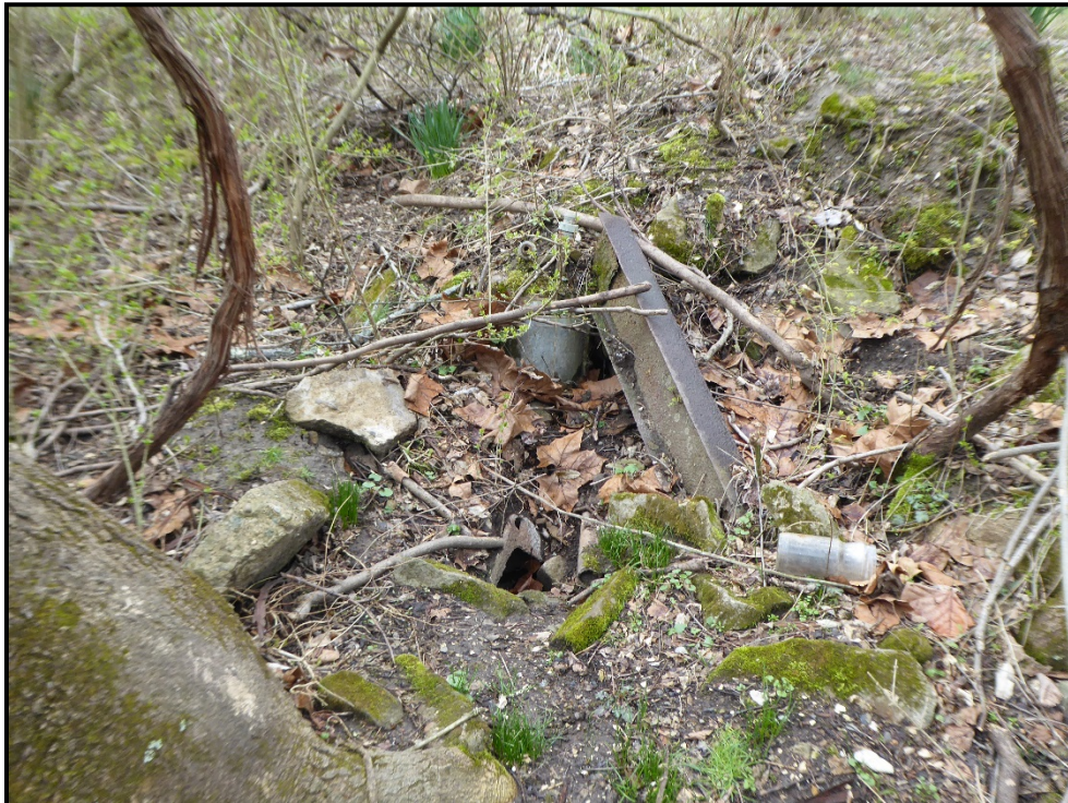
Figure 38: Rubble within the foundation.
