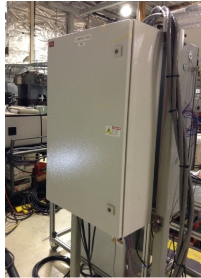
Data acquisition panels
