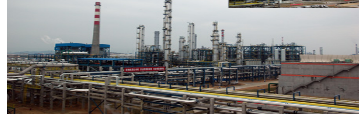
Yangtzi Petro-chemical Plant
