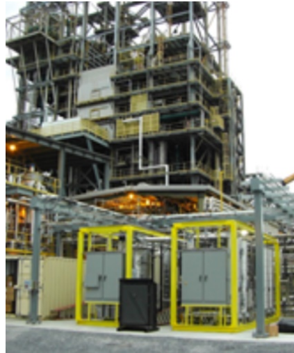
TDA 0.1 MW pre-combustion carbon capture unit installed at the National Carbon Capture Center
