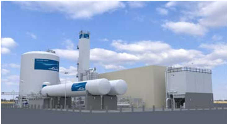
Linde Air Separation Plant ( www.linde-engineering.com )
