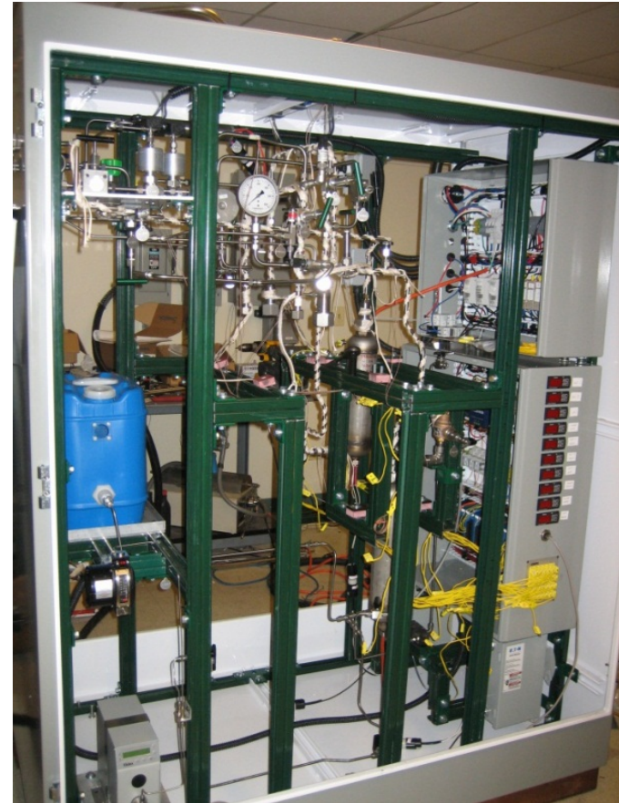
Gas Conditioning Skid
