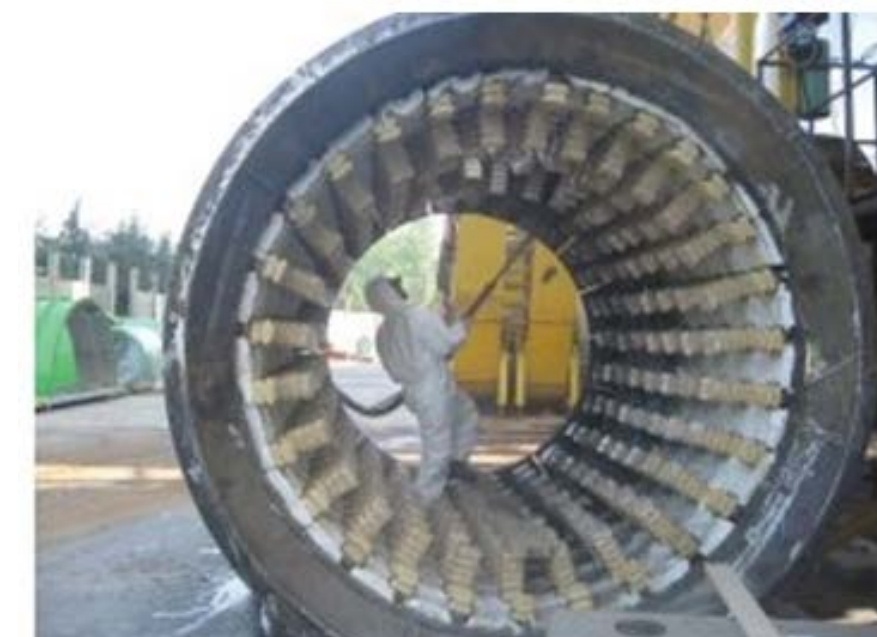
Anchors (left, image from TFL Houston) might be installed using powder feed or wire feed AM, while gunning (right, image from Kiltas) might be controlled via robotics.
