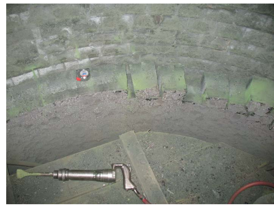
Traditional Gasifier Liner Removal/Rebuild
