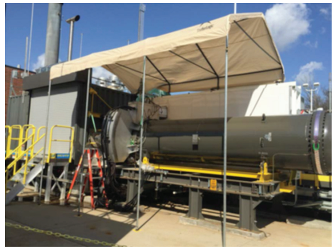
Figure 3. Photo courtesy LG Fuel Cell Systems
